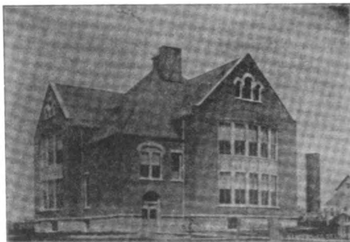
NORTH SCHOOL BUILDING, LANCASTER.
